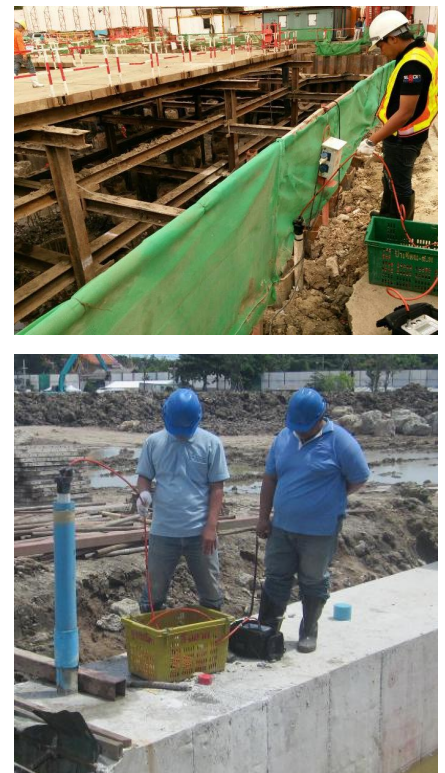
Fig. 4 inclinometer reading on site
