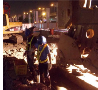
Fig.9 Example of application measure the actual lateral movement of soil near underground tab water tunnel during Barrette pile construction. Measured data of each step are calculate immediately and present on site, continuously 72 hrs.
